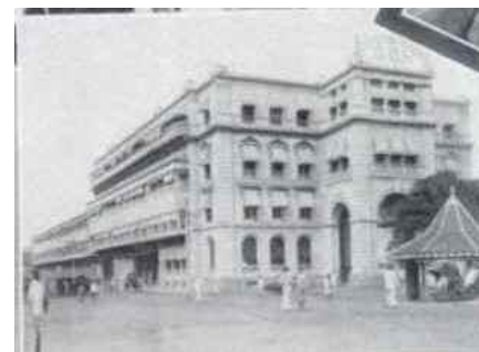
GOH Building (Now Hotel Taprobane)
